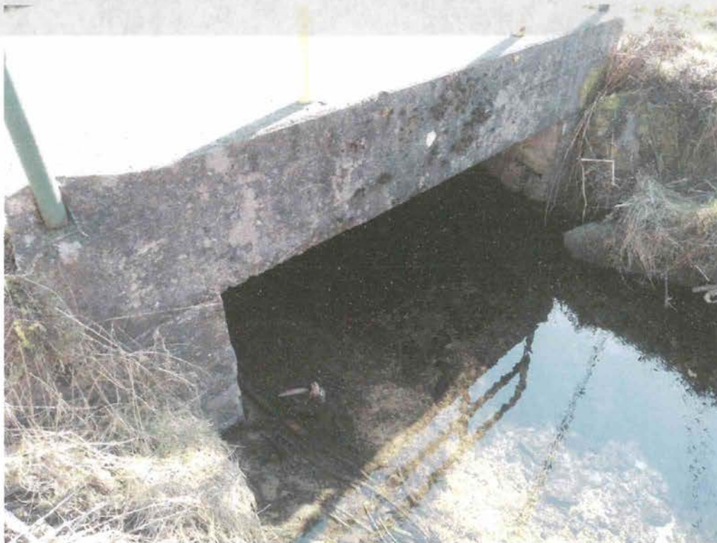
4 – Pont DALLE Elevation aval
